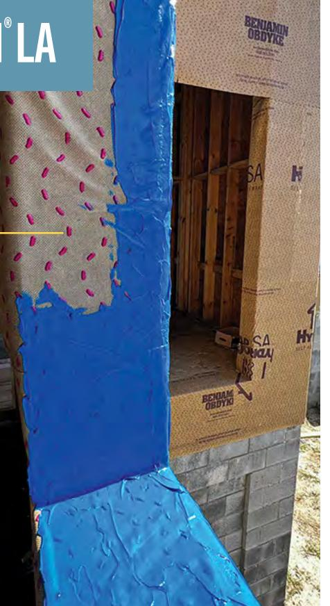
use for challenging details in exterior insulation applications, including geometrically challenging areas
