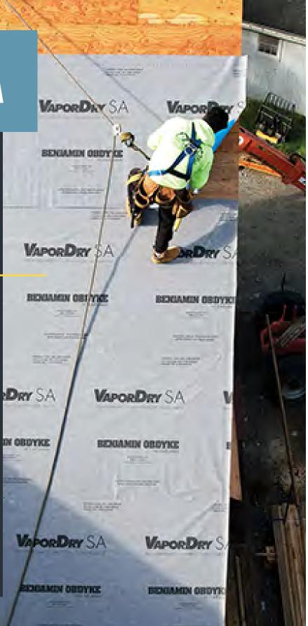
use with cedar breather for maximum drying potential in wood & metal roof applications
