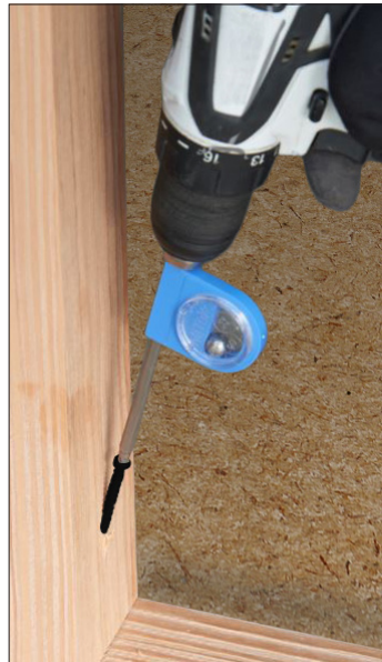
Typical WSTS45-EXT stud to bottom plate installation
