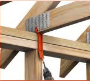
DOUBLE TOP PLATE TO TRUSS
