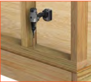
BOTTOM PLATE TO RIM BOARD
